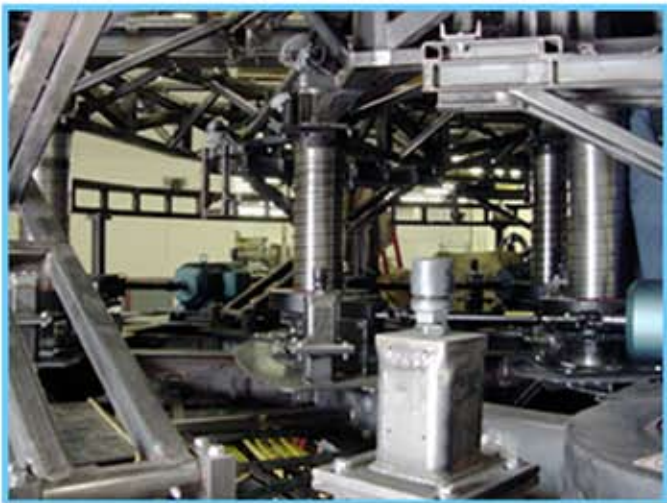
STAGE LIFTS & TURNTABLE (SHOWN DURING FABRICATION)
